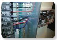
Series TSni100 - Non-Modular SPD Mounted with Direct Feed from Panel Breaker
