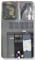
Series TSri300 Modular SPD Mounted on Top of Service Entrance Switchgear; Bottom Feed Configured
